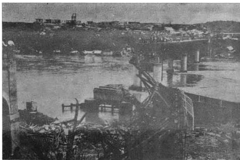
Puente "Ozama". / "Ozama" Bridge.
